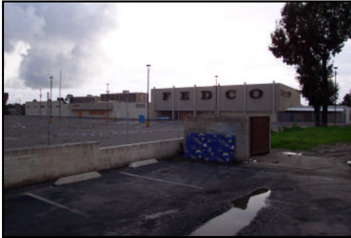
Photo 1: Photograph of vacant 140,000 square foot Fedco department store building. The 30-year-old structure is undersized and needs to be demolished to be useful for future anchor tenant use.
