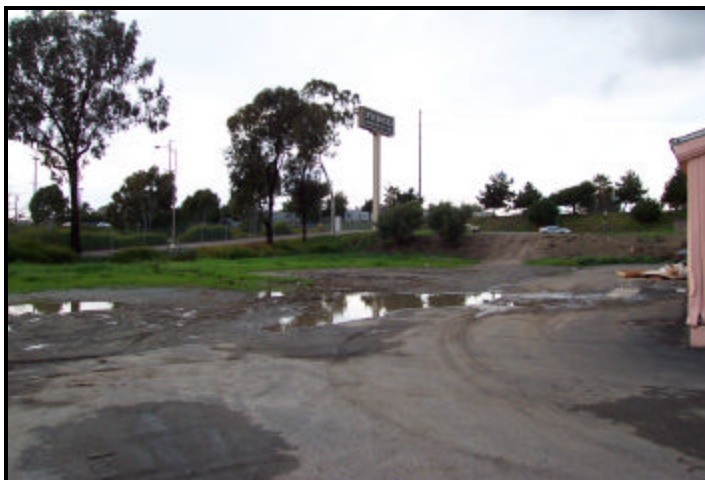
Photo 3: Unpaved, submerged portions of the smaller commercial properties near the intersection of Plaza Boulevard and Highland Avenue. These
